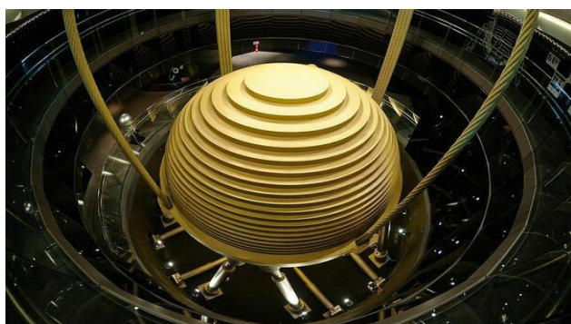
Figure 10 Tuned Mass Damper
